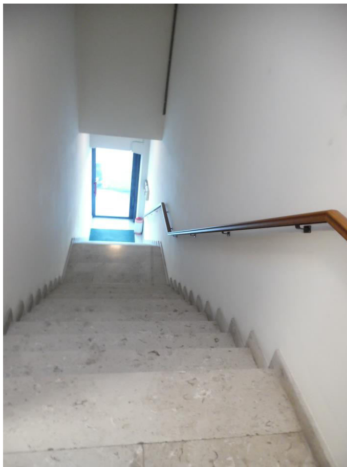
Vano scale – Sub. 63
